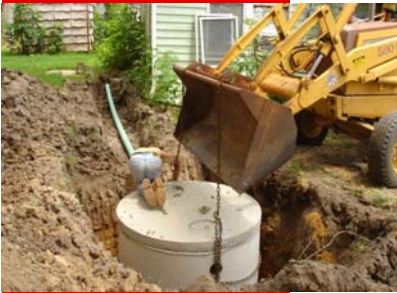
Installing a rural Waste Water System in Brazos County.
